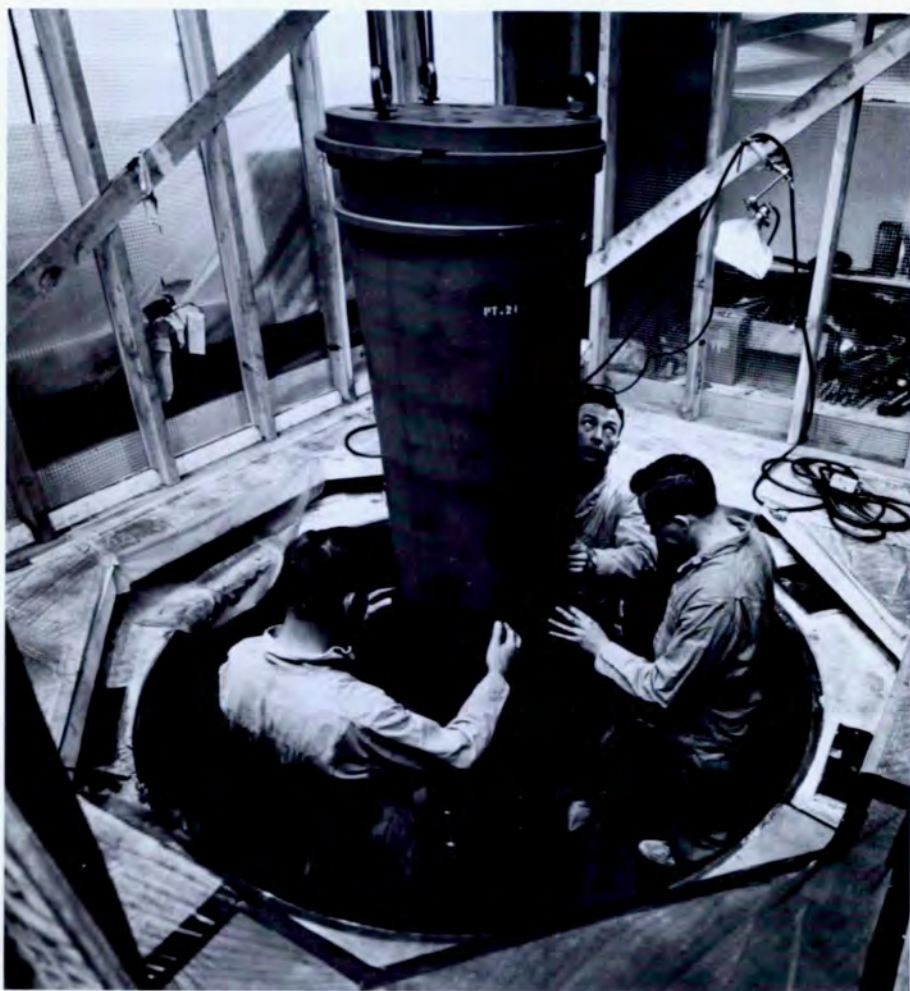
The UHTREX reactor core being lowered into its containment vessel.
